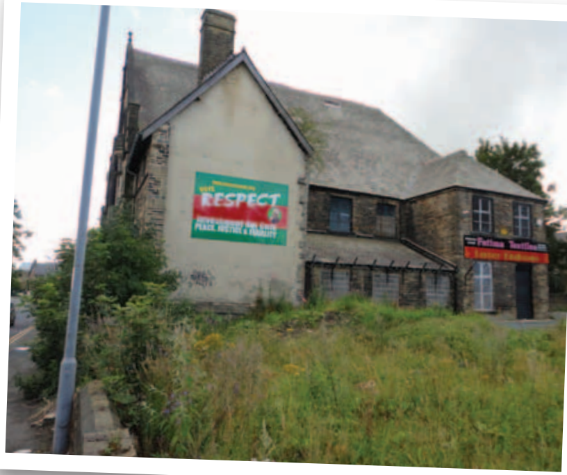
Derelict building in Manningham
